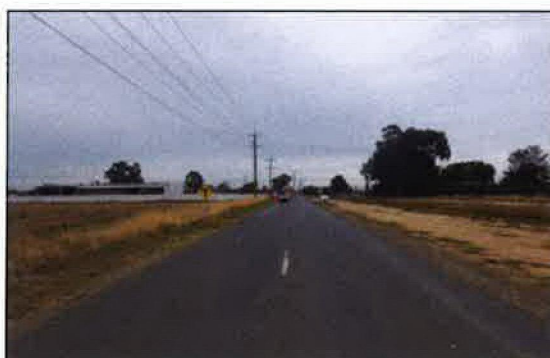
Figure 10: Ford Road view West
