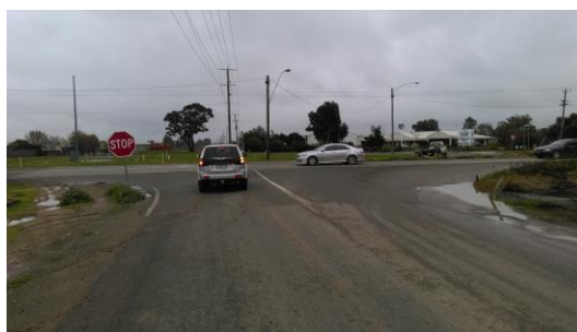
Figure 2.6: Ford Road (looking west)
