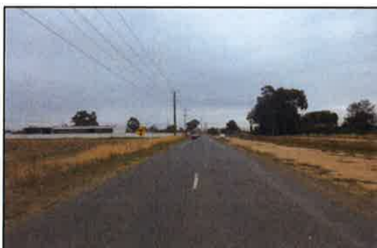
Figure 10: Ford Road view West
