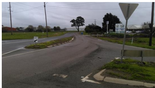
Figure 2.8: Wanganui Road (looking west)
