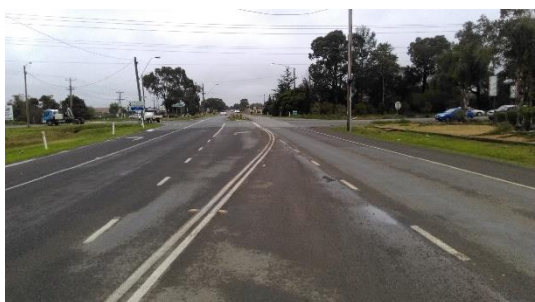
Figure 2.1: Goulburn Valley Highway (looking north)
