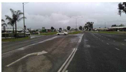
Figure 2.2: Goulburn Valley Highway (looking south)
